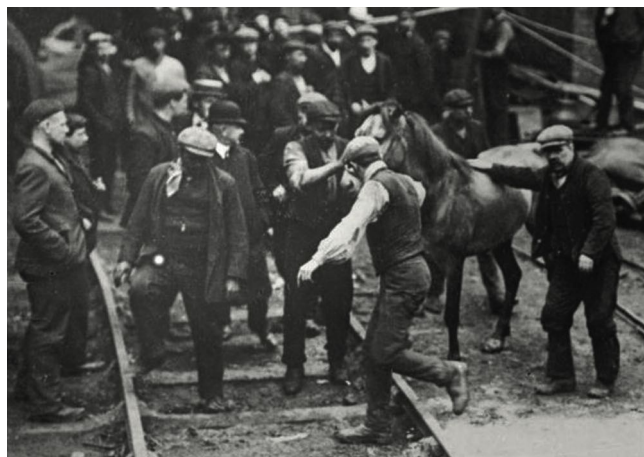
Bringing up the pit ponies after the 1908 Maypole colliery explosion
